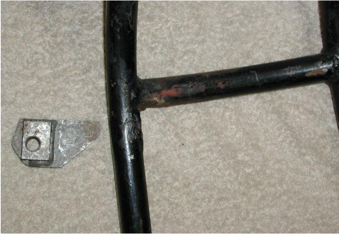
A picture of the frame with the old bracket removed and the a new bracket to be installed.
